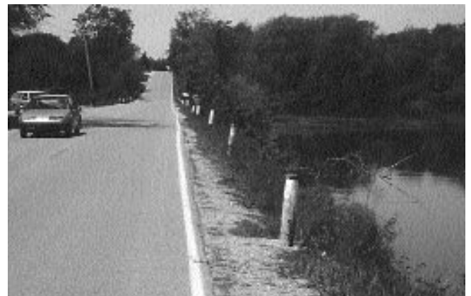
Deep water at the bottom of a steep slope can be dangerous.
