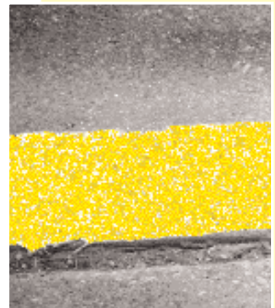
Above: Using glass beads on pavement markings improves visibility and gives skid resistance for pedestrians.
