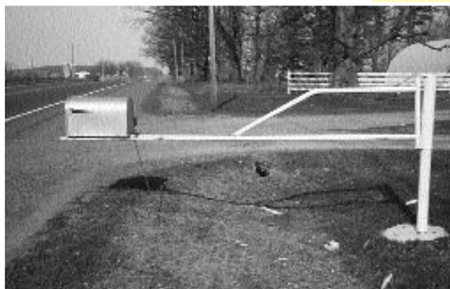
Bottom right: Good installation. Post is set back from roadway and mailbox is firmly attached on a swing-arm system.
