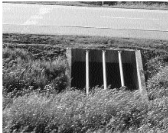
Bottom right: Concrete culvert opening protected with steel grating improves safety.
