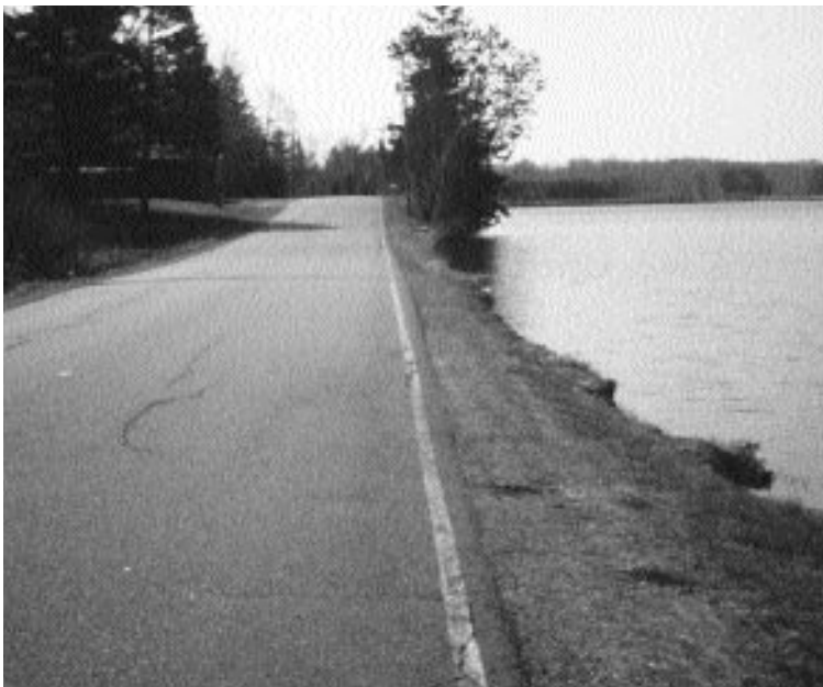
Left: Edge of shoulder could be delineated with water reflectors to mark water hazard. Guardrail could be used if warranted by accident data and experience.
