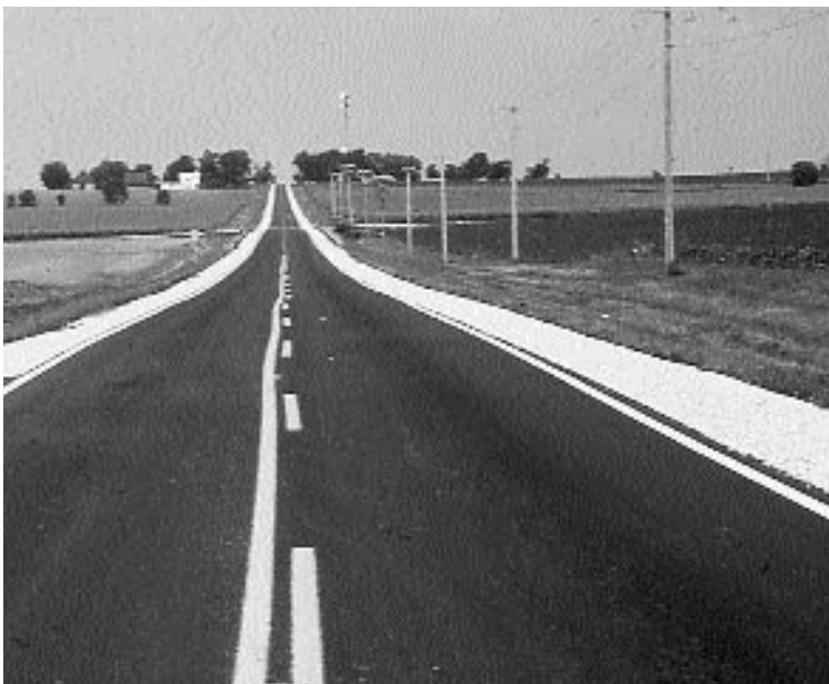
Good geometrics with adequate lane and shoulder width.
