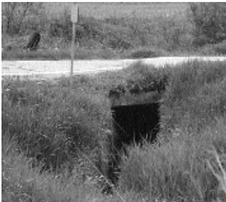
Large dropoff at culvert located very close to edge of roadway is dangerous.
