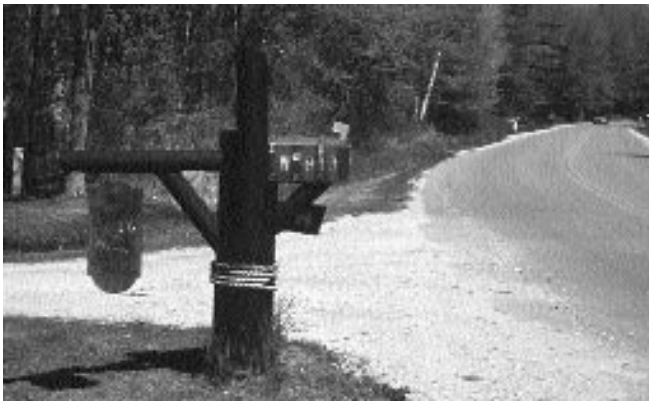
Hazardous mailbox support using telephone pole.
