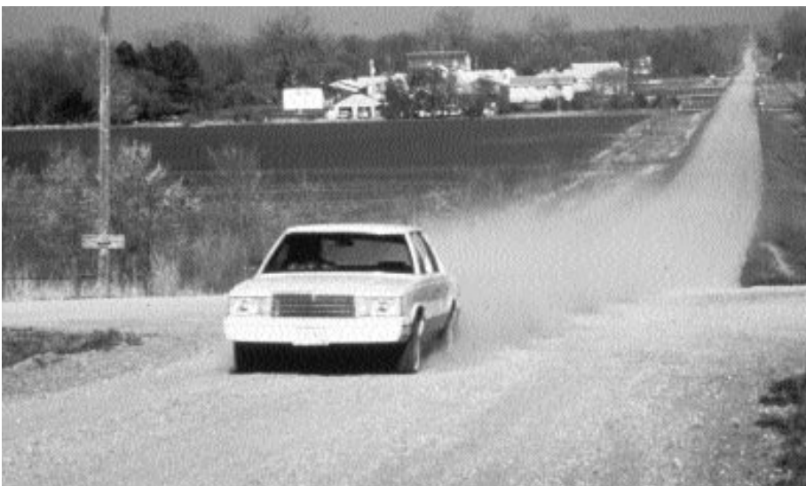
Bottom: Narrow and unsurfaced roads can provide an adequate and less costly level of service on lower volume roads.
