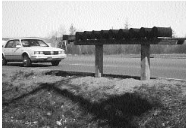
Installation of mailboxes on plank is dangerous. Plank is at height that would allow it to penetrate into the vehicle's passenger compartment.
