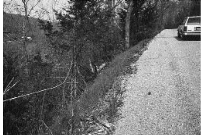
Steep slope will carry vehicle down to hazardous trees.
