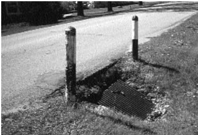
Large dropoff at culvert located very close to edge of roadway is dangerous.
