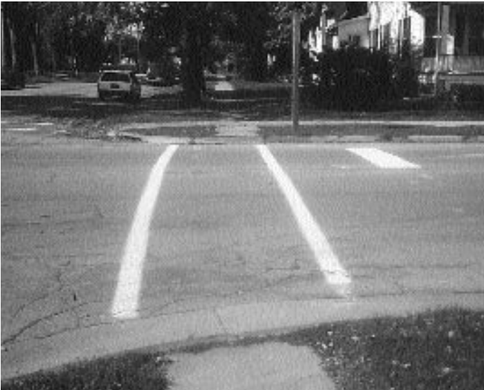
Narrow crosswalk. Proper stop line.
