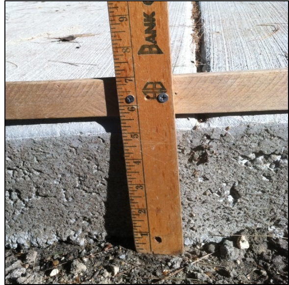
Figure 34: Five inches of concrete sidewalk
