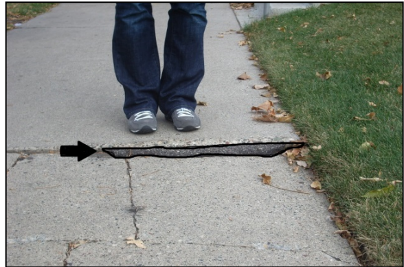
Figure 24: A small wedge may still create a hazard or be difficult to navigate in a wheelchair. This wedge had deteriorated over time.
