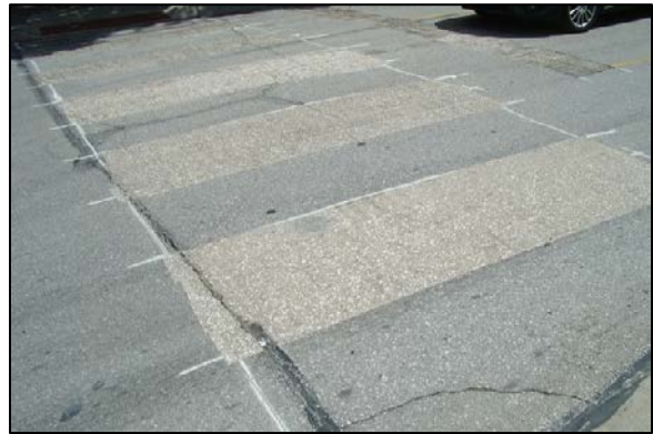
Figure 32: Old crosswalk markings removed for new crosswalk marking tape.
