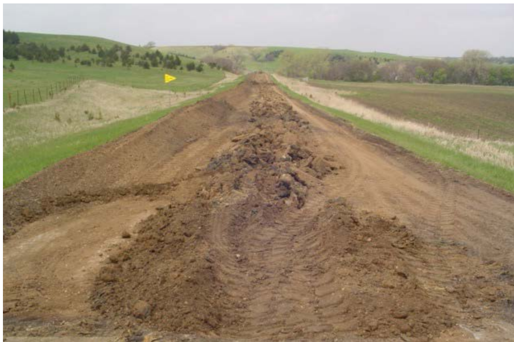
A road that had a constant problem with water percolating upward from springs beneath the surface. Work has just been completed to plow drainage pipe into the subgrade of this road.
