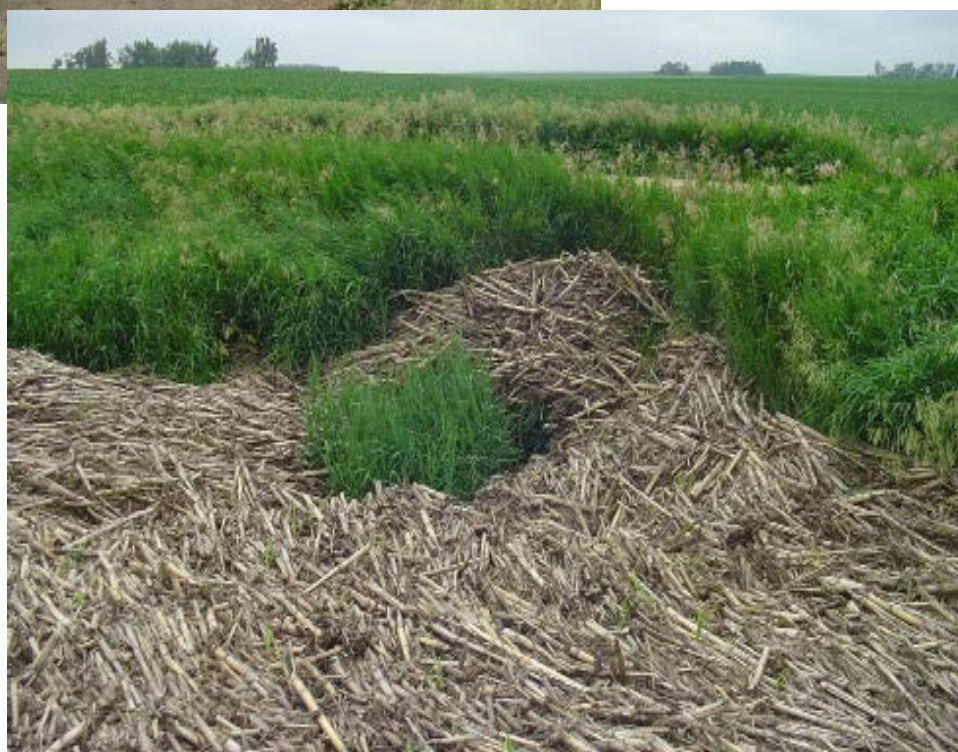
This road could fail if debris is not cleared before the next heavy rain.
