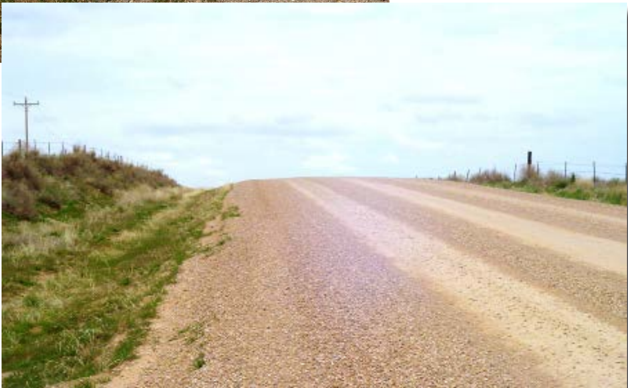
These photos (left and below) show good examples of gravel shoulders that match the edge of the roadway very well and drain water to the ditch.
