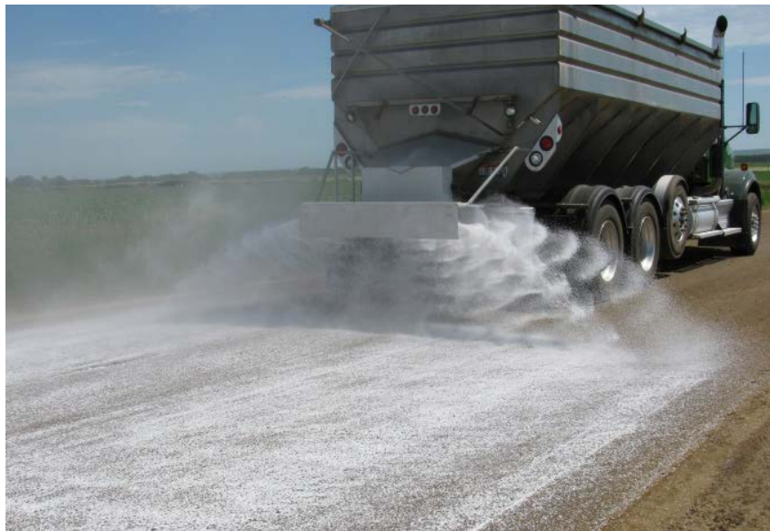
Good example of even application of chloride in dry form – cannot be done in windy conditions.
