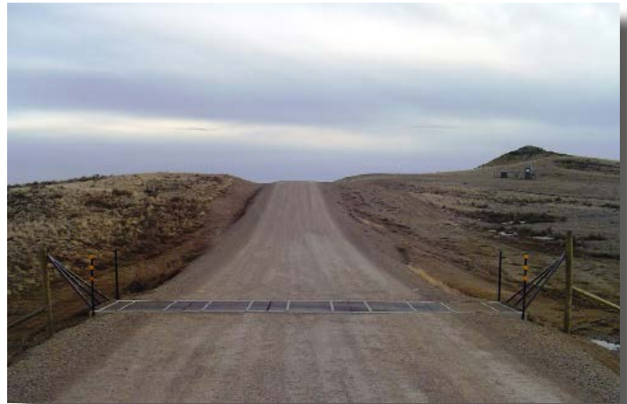
Road is shaped very well for a smooth crossing over the cattle guard.
