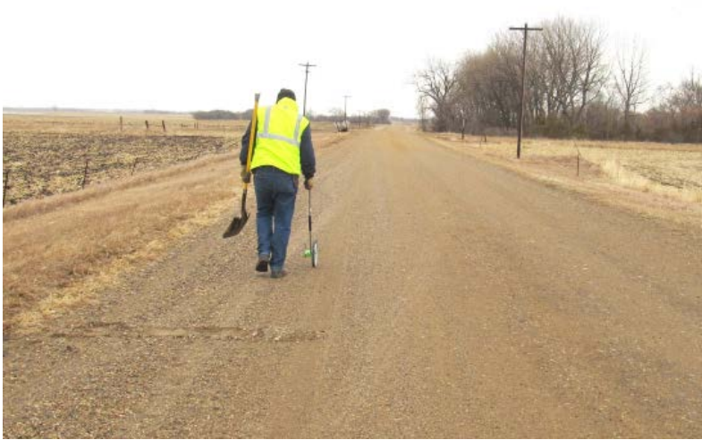
A very good practice of measuring and marking spread distance for incoming trucks with a measuring wheel and shovel to make a mark on the surface.
