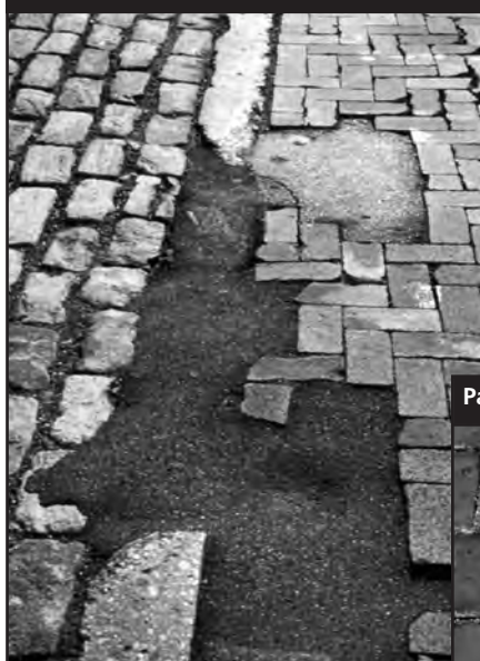
Patches for missing bricks and blocks.
