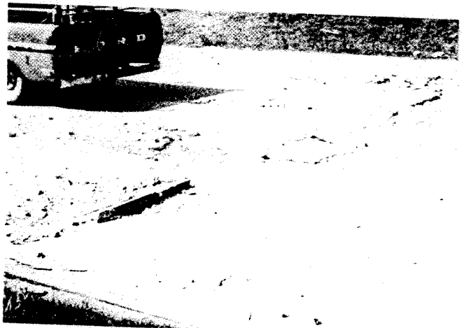
Police, solid waste collectors, utility workers—every municipal employee—should watch for defects like this pavement blowup.
